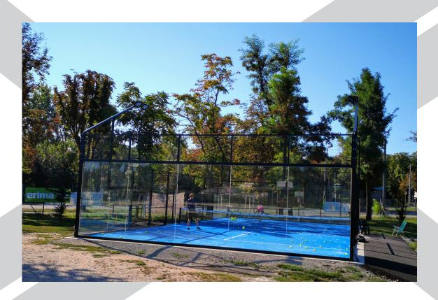
International tournament court design – all glass panels 3m height tempered security glass 12mm, 3mm steel frame, zinc treatment and powder coated finish MONDO (LOGO) STX90 padel turf, LED flood lights
